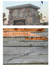
BOARD FORMED CONCRETE PILASTER AND PRECAST CAP
