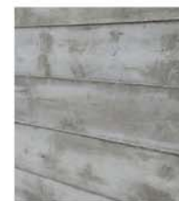
BOARD FORMED CONCRETE PILASTER AND PRECAST CAP
