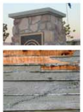
BOARD FORMED CONCRETE PILASTER AND PRECAST CAP
