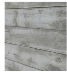
BOARD FORMED CONCRETE PILASTER AND PRECAST CAP
