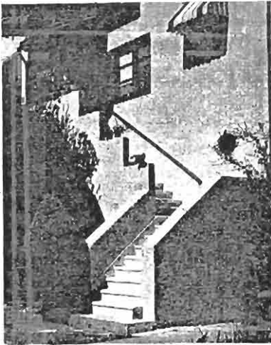
ILLUSTRATION OF STEPPED STAIR RAIL The use of the stepped stair rail is very ancient, it is found in Roman ruins. Note also the mid-landing, turned stair and the shortened rail on one side to expose the lowest stair riser. (Architect and source unknown)
